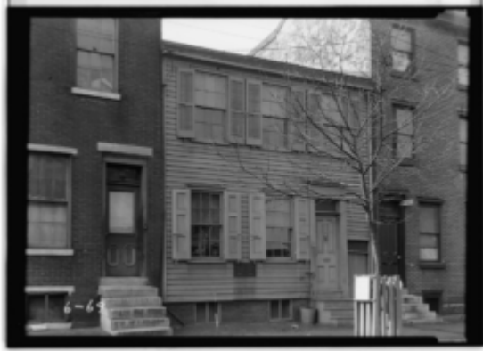
Figure 1: Walt Whitman House, 328 Mickle Street, Camden, Camden County, NJ Historic American Buildings Survey. Nathaniel R. Ewan, Photographer April 15, 1936/ Library of Congress
