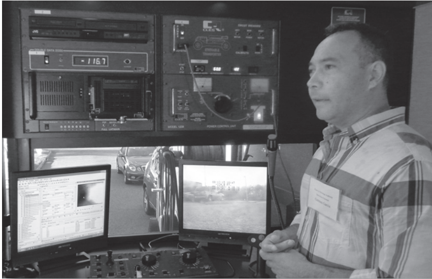
Germain Garcias discuss the CCTV inspection system that Township of Hanover SA uses as part of its asset management program.
