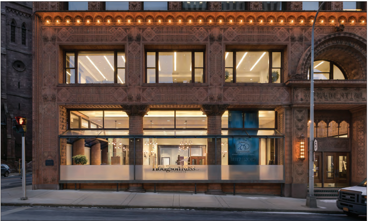
Hodgson Russ embarked upon an extensive renovation of the Guaranty Building beginning in 2006. The project would eventually include the restoration of the building's elaborate terra cotta exterior, and would provide the firm with a breathtaking home for their third century of existence. © 2017 KIM SMITH PHOTO
