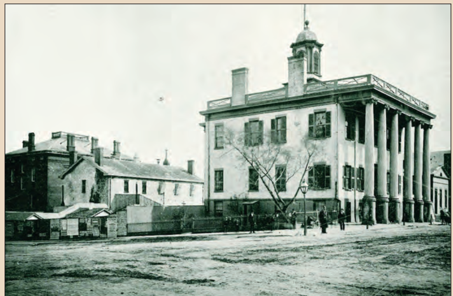
The Erie County courthouse, ca. 1898. Finished in 1817, the structure was located where the Buffalo and Erie County Public Library now stands. Asa Rice’s 1822 law office was located nearby. WESTERN NEW YORK HERITAGE COLLECTION
